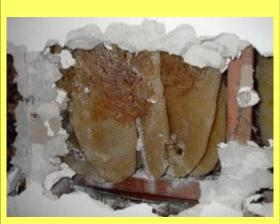
This is a photo of what honey comb looks like inside the wall of a house. In this instance the bees came in a hole from the outside and made their bee hive between the two studs underneath a window. This shows the plaster board broken away after the bees had been disposed of.
